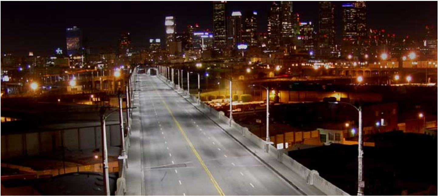
6th Street Bridge, Los Angeles uses 100 LED, Type II LEDway units
