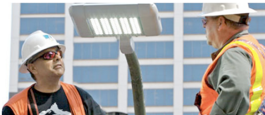
PG&E workers installing an LED streetlight. Photo: PG&E
